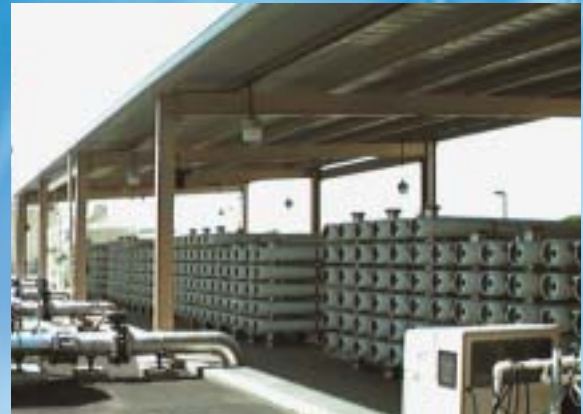
ESPA installation, 5 MGD, in Carson, California
